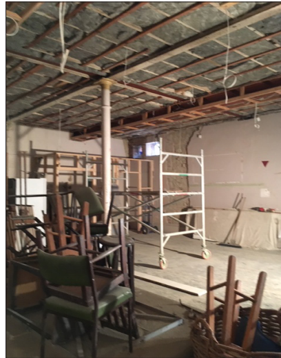
Studio with the ceiling missing
