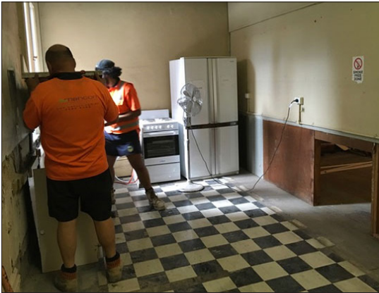
Kitchen being demolished
