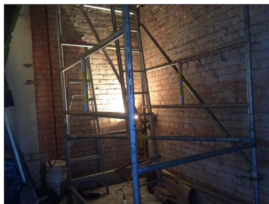
Bricks cleaned back to original state in Hammond storage space
