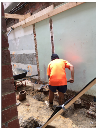
The old toilet block
