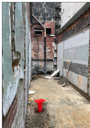
The old toilet block
